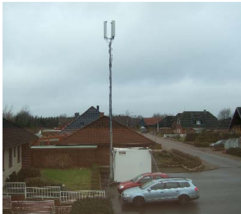
Abb. 23 Teststation in Sillerup
